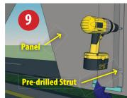
Step 9—Drill and Fasten Panels Drill the panels using the pre-drilled struts as a guide. Use a 17/64" drill bit.
